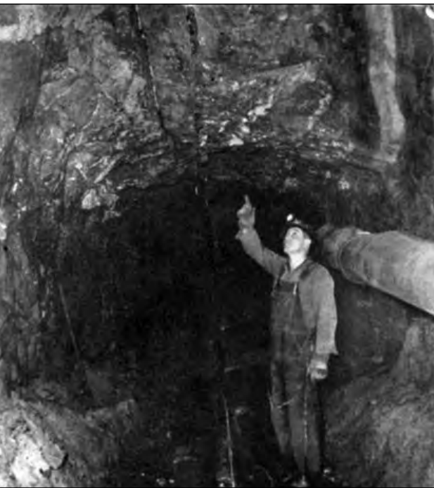
Dixie Martin, mine foreman, points to one of the underground fault lines. The other fault line follows the light band visible above on the right.
